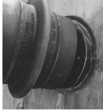
3. Place the Century-Line® Sleeve on the end cap. The sleeve and endcaps total length should be one-fourth longer than the width of the wall. Cut with a hand or power saw.
