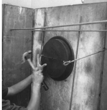
2. Nail one of the end caps at the marked center line.
